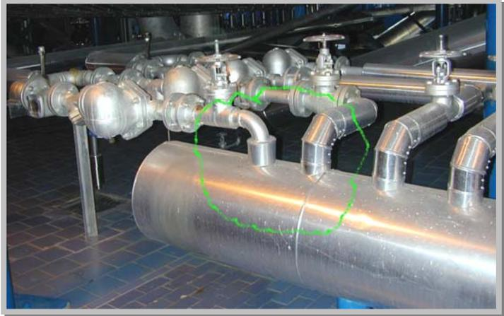
\* Picture indicates the proper connections to the main condensate header.
