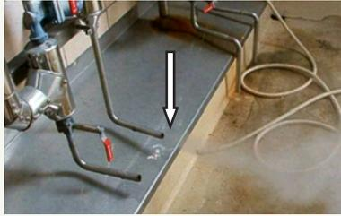
Picture number 2 shows the discharge from the valve off the steam line to be very visible with liquid being discharged with the steam vapor.
