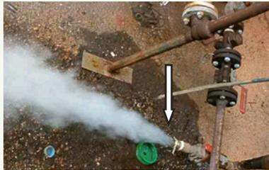
Picture number 3 shows the discharge from the valve off the steam line to be very visible with liquid being discharged with the steam vapor.
